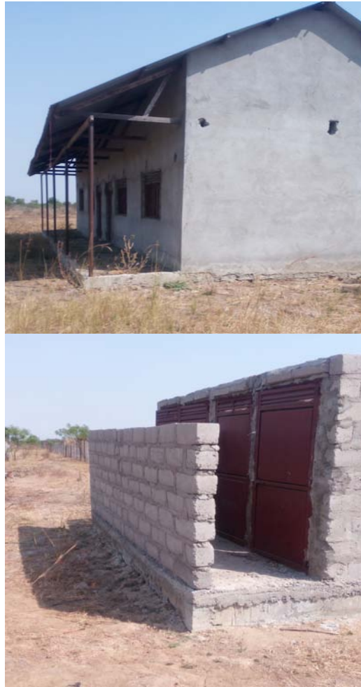
Classroom and toilet block nearing completion
