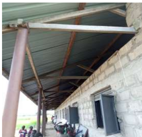
Upper sections of brickwork were repaired last month
